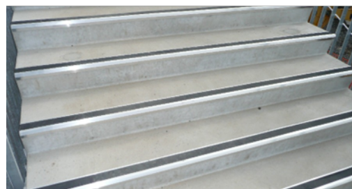
Concrete Finished Stairs
